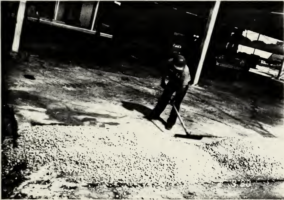
Figure 2.5 Leveling Off Coarse Aggregate
